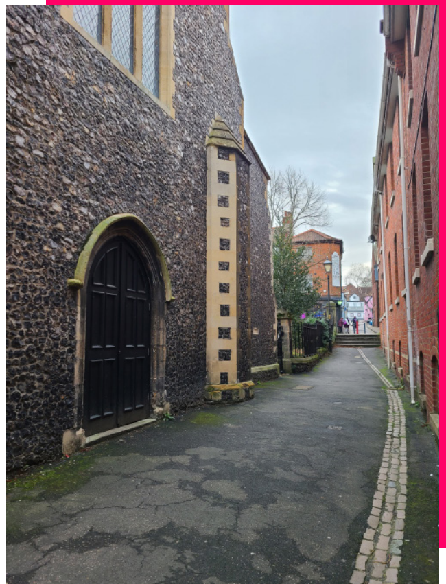
LOAD IN DOOR
